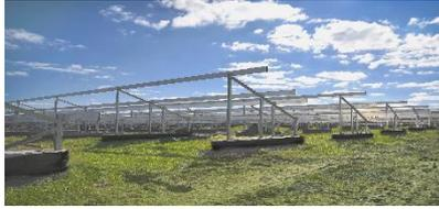
The L&D Landfill 12.9 MW GameChange Racking Pour-in-Place™ System is the largest superfund landfill project in the United States.
