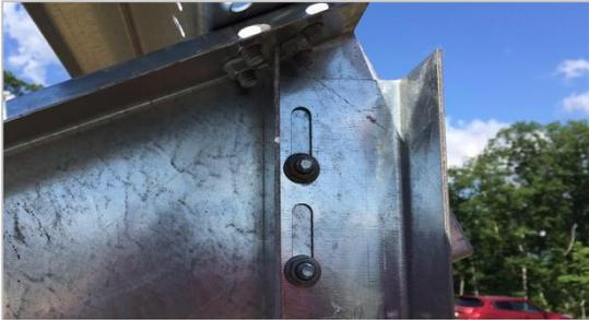
Slots combined with rail support self-leveling technology enable up to 10" vertical adjustability
