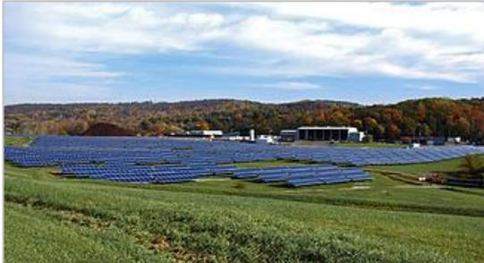
East-west slopes up to 15% for continuous systems no ground prep required. North-south slopes up to 5% need no gravel buildup under forms, over 5% up to 15% need buildup
