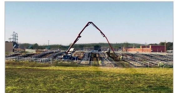
Standard concrete pump truck has long range and fills up to 2.5 MW of Pour-in-Place™ forms per week
