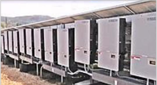
String inverters and homerun wiring attach easily to Pour-in-Place™ System
