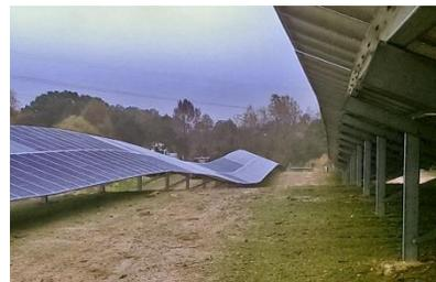
Articulating purlins between tables enable installation on sites with complex slope issues including up to 15% east-west terrain slopes
