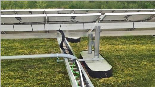
North-south wire management trays for homerun wires mounted on Pour-in-Place™ system
