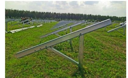
Nesting components eliminate brackets, have long slots enabling three axes of adjustability
