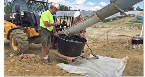
Gen4 Pour-in-Place™ Ballasted Ground System with round forms shipping Q4 2015: no temporary bracing, less concrete, faster install, steeper slopes up to 17% in all directions
