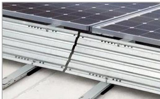
Pre-punched slots in wind defectors enable fast east-west string wiring prior to panelizing
