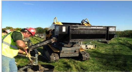
Pouring bucket on bobcat for concrete pouring of Pour-in-Place™ forms on sensitive landfill caps
