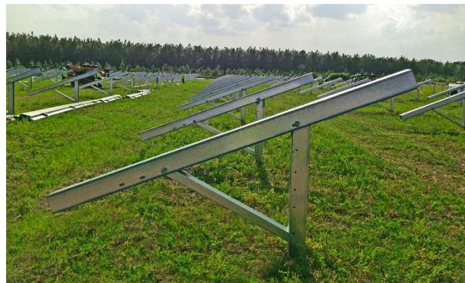
Nesting components eliminate brackets, have long slots enabling 3 axes of adjustability
