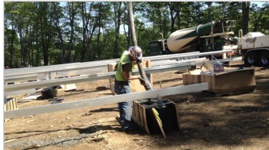
Filling Pour-in-Place™ forms using concrete pump
