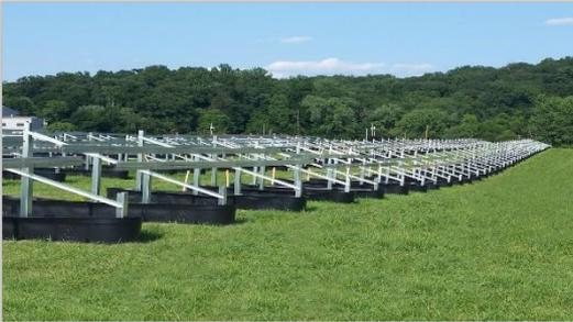
Place supports, attach rails, then level rail supports quickly prior to pouring concrete
