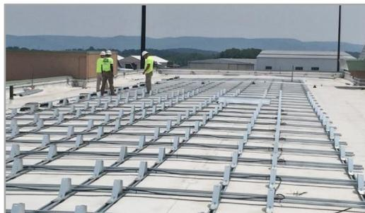
Interlocking grid design combined with NextGen wind deflector virtually eliminates ballast to minimal or zero
