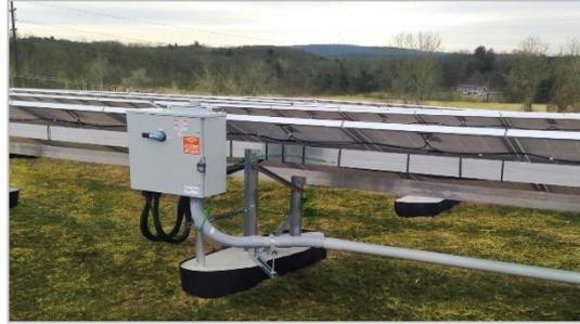
Combiner boxes and string inverters mounted on to support structure in Pour-in-Place™ forms
